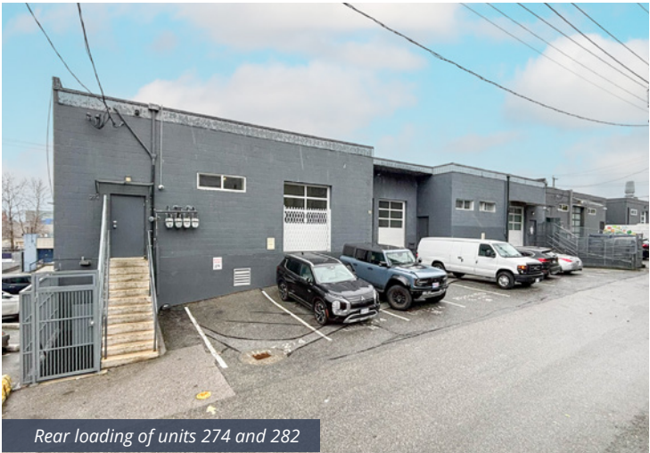
Rear loading of units 274 and 282
