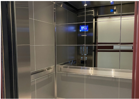
Complete elevator cab retrofit with flush mounted LED screens
