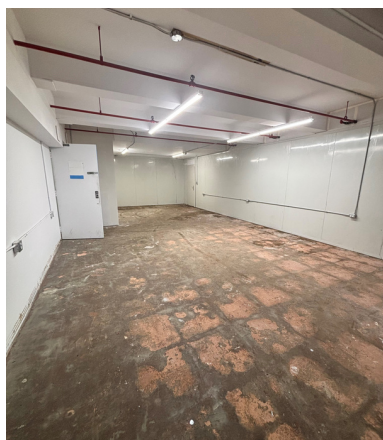
Lower Ceiling Section
