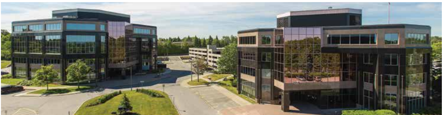
Qualicum Centre office complex
