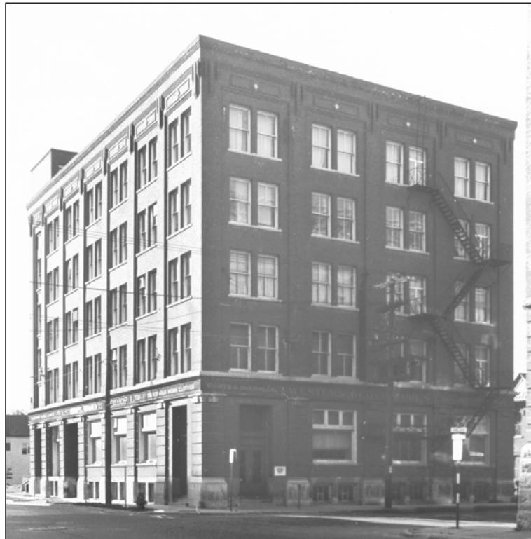
Plate 4 - Western Glove Building, 321 McDermot Avenue, 1970. ( Courtesy of the Provincial Archives of Manitoba, Architectural Survey. )
