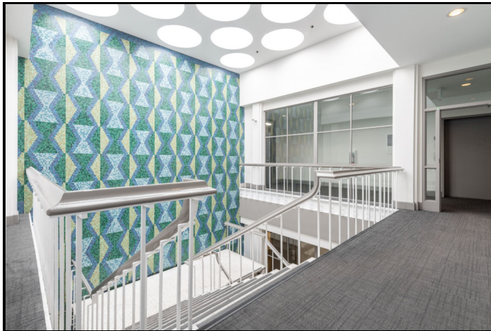
SECOND FLOOR MAIN ENTRANCE:
