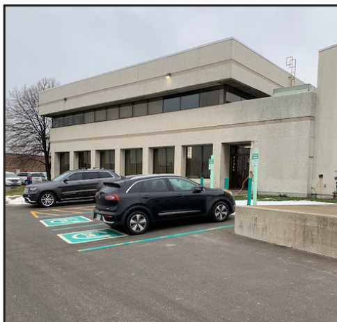
East Side Building
