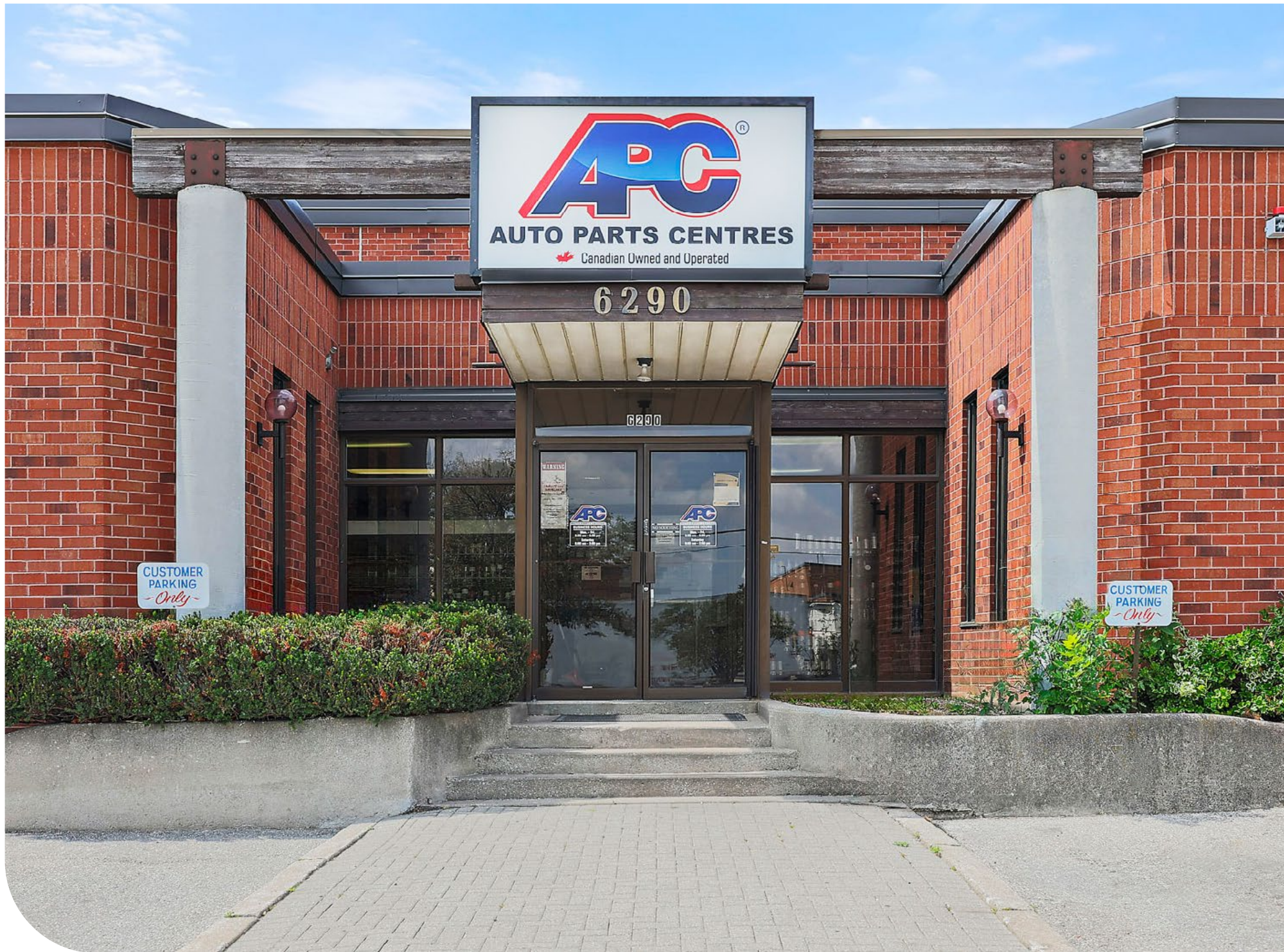
4 6290 KESTREL ROAD, MISSISSAUGA, ON
