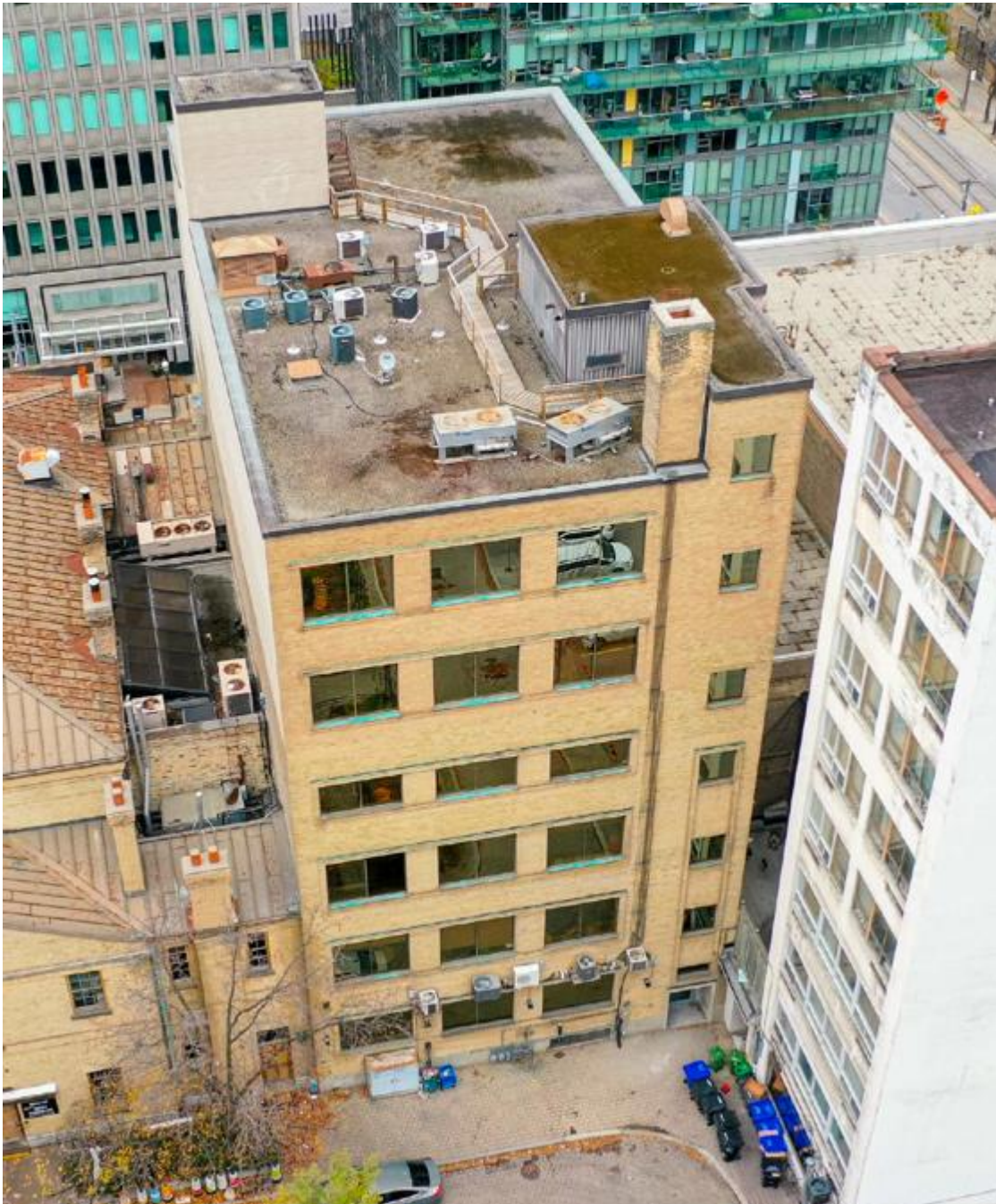
Court Street view
